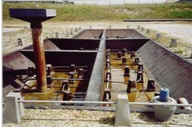
When the submersible pump is started at least a well plus surface plant volume is pumped to the sea through a methane degassing and sedimentation sewage pipe buffer basin
